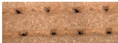
No TiO 2 particulate migration through stitch holes of the seam taped filter bag after 18 months of service.
